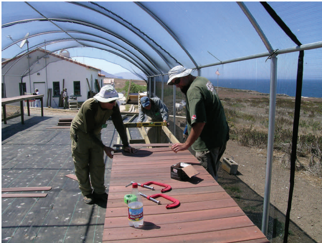
CIR personnel construct Anacapa Nursery 2010
