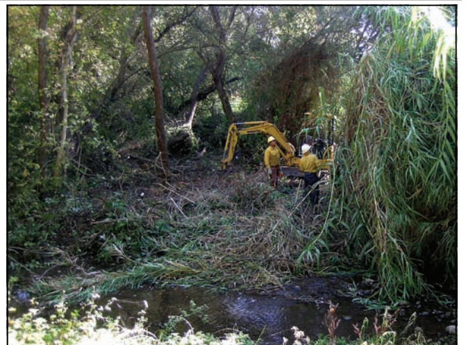
Arundo removal near the Santa Ynez River
